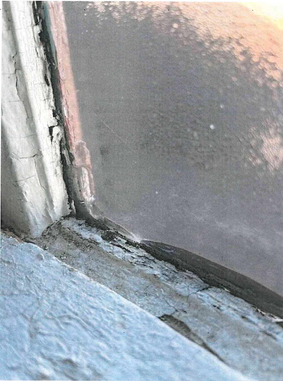
Window in bedroom that is safety issue because of height from floor.
