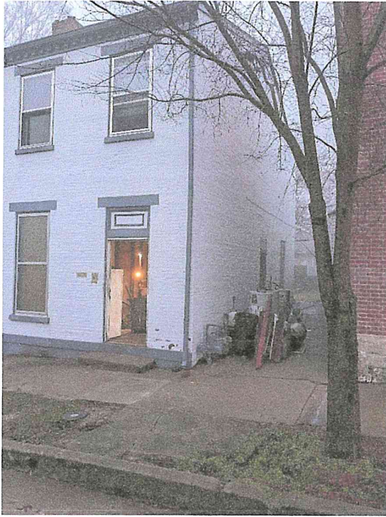
Doors not visible from street Front Windows to repaired and painted
