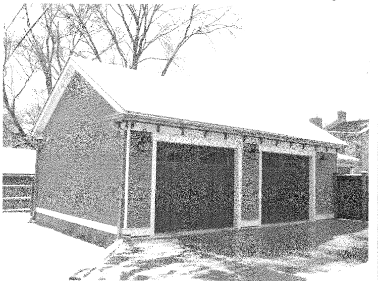
YES: The new garage at 513 Mulberry Street was designed to be compatible with the new primary dwelling through its gable roof, weatherboard siding, and paneled garage doors.
