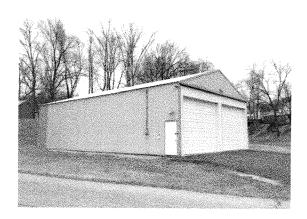
**Description/Remarks**This is a 1-story garage built in 1990. The foundation is not visible. Exterior walls are metal. The building has a gable front roof clad in standing seam metal. Side metal door with two front garage doors.
