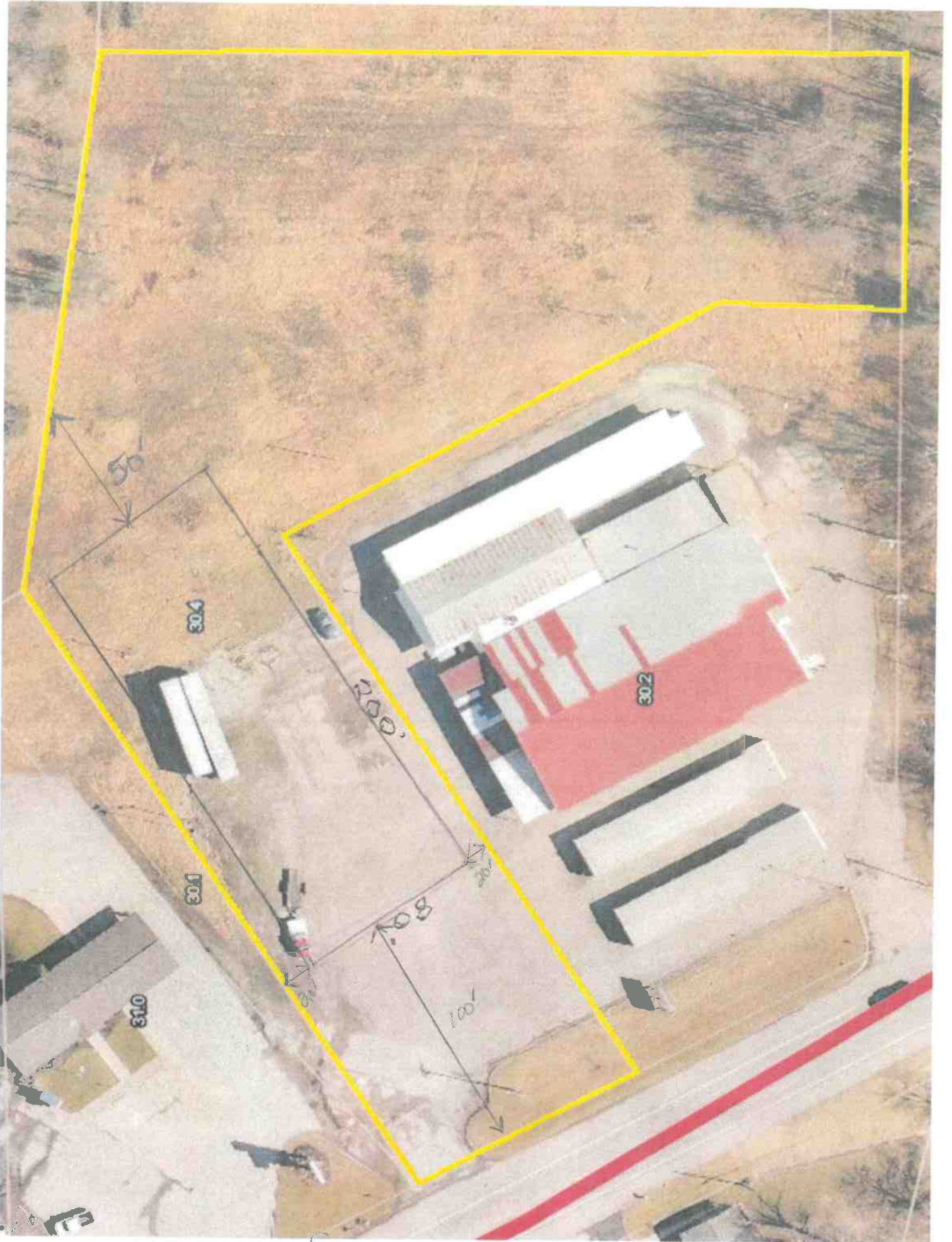
Lanier Drive Retail Building & 10' Road
