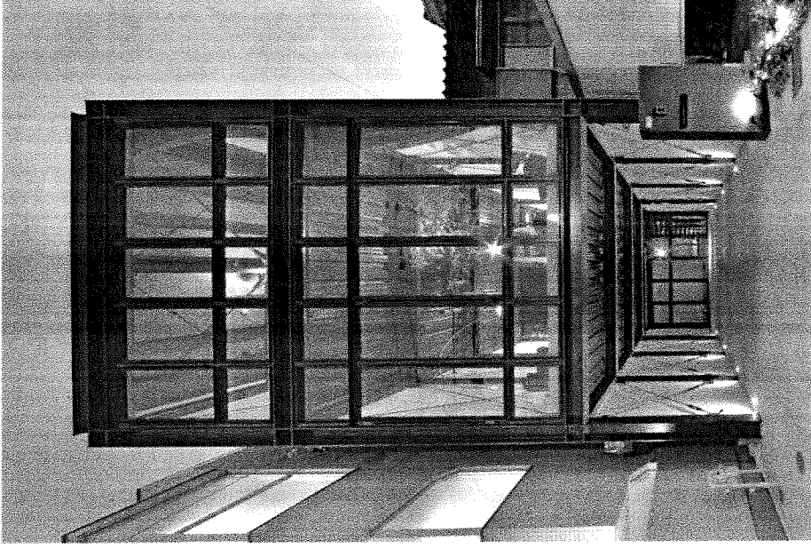
Future Conceptual Design- lower level open patio Story 1 & 2 closed in glass rear with metal roof, steel/wood structure
