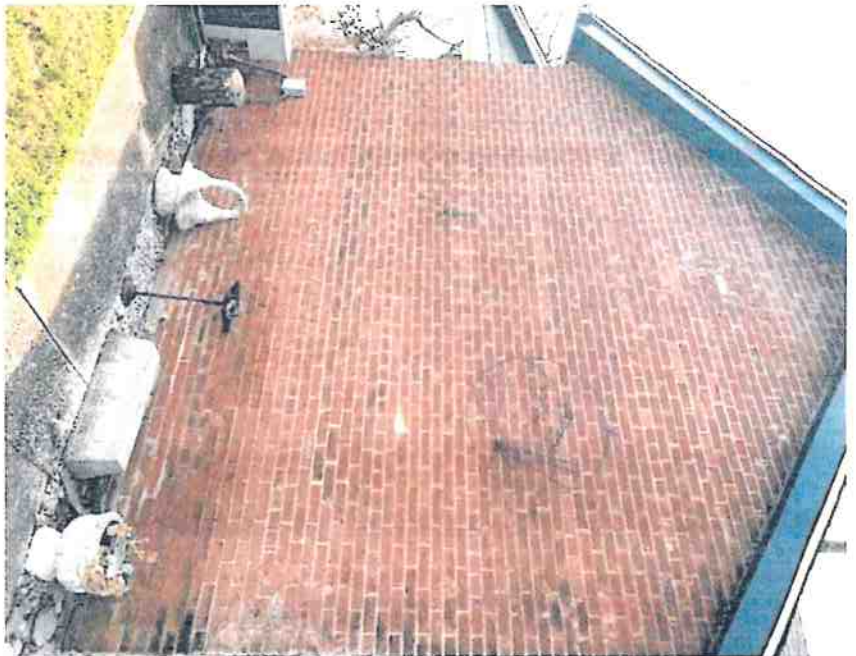
East wall original
