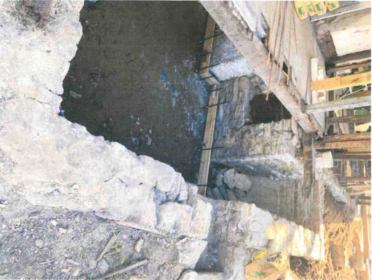
Stone foundation repair
