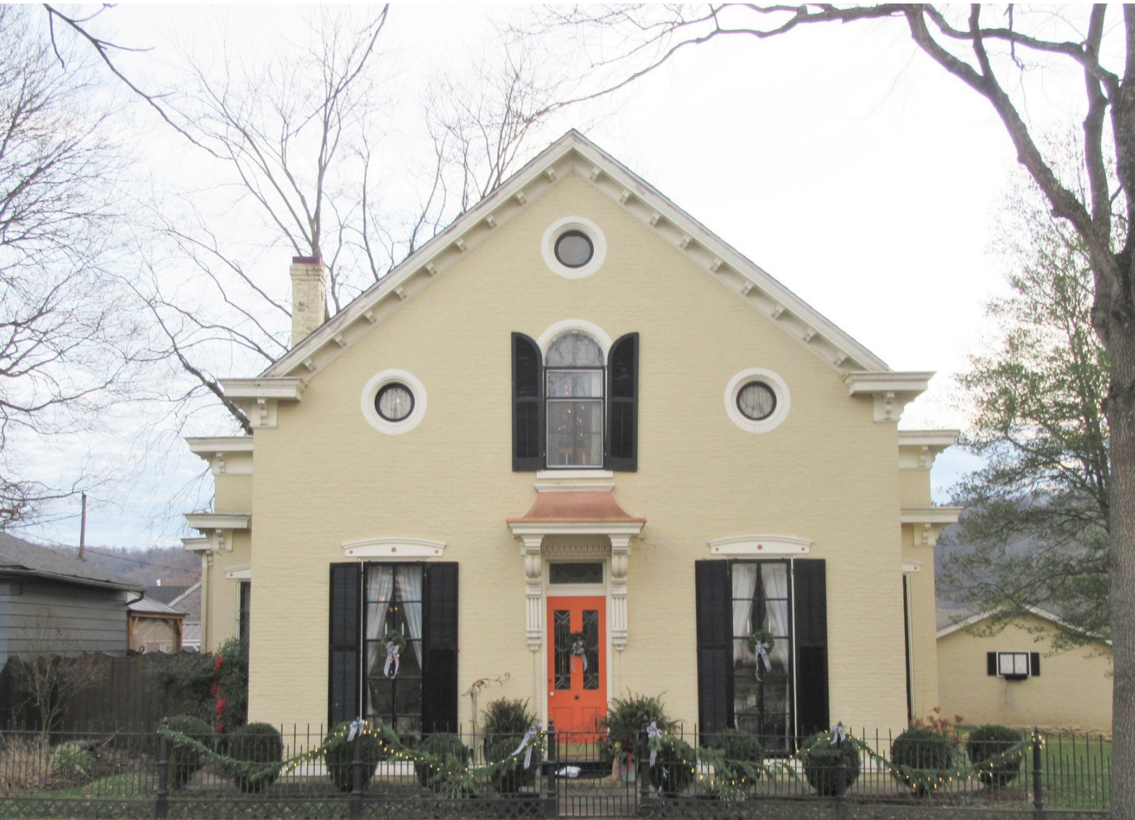
Stribling House, 625 W. 2nd Street
