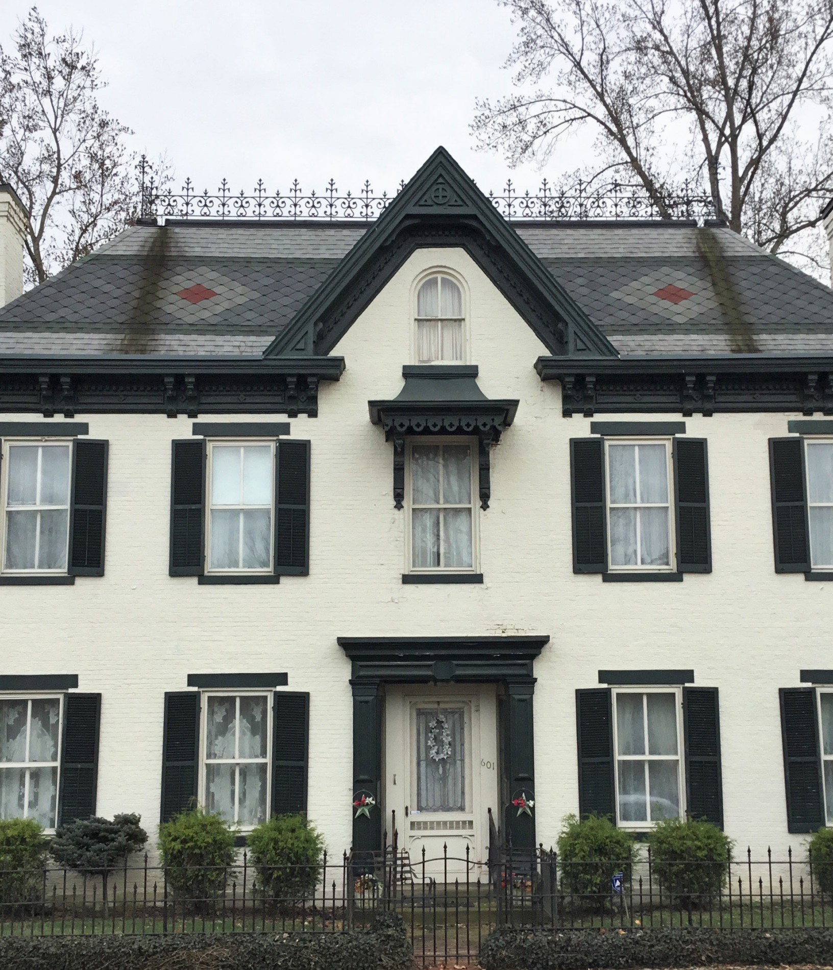
Crawford House, 601 W. 2nd Street
