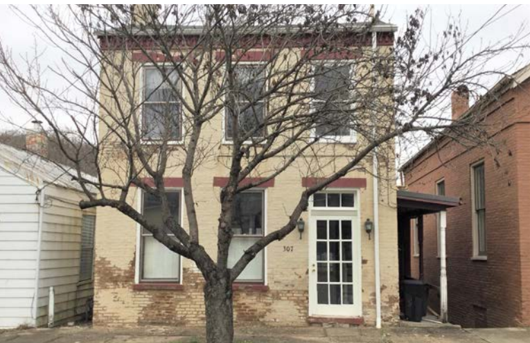
William Douglass House, 307 E. 5th Street
