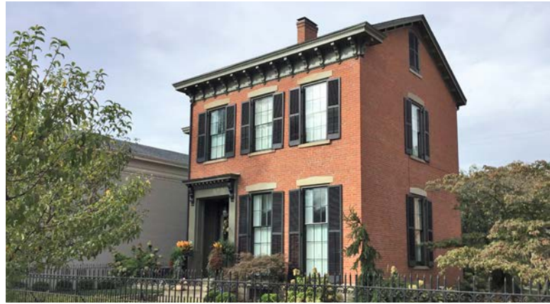
416 W. Main Street (2/3 Single Pile)
