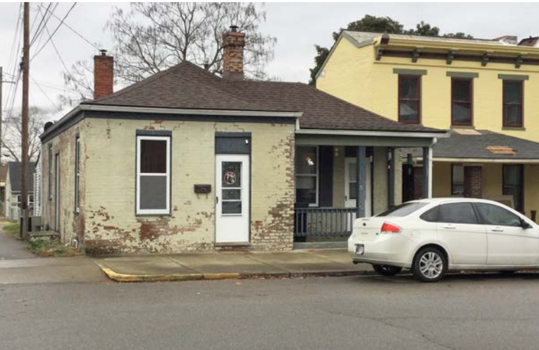
Stafford House, 619 Walnut Street
