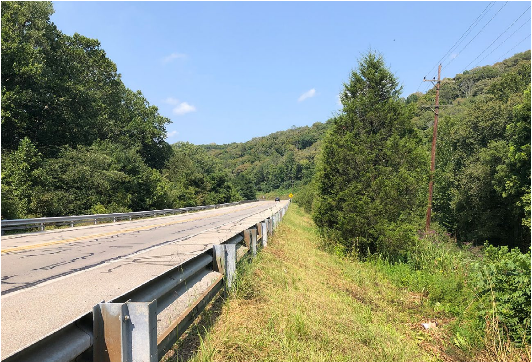
VIEW 01 | BRIDGE OVER CROOKED CREEK EXISTING CONDITION
